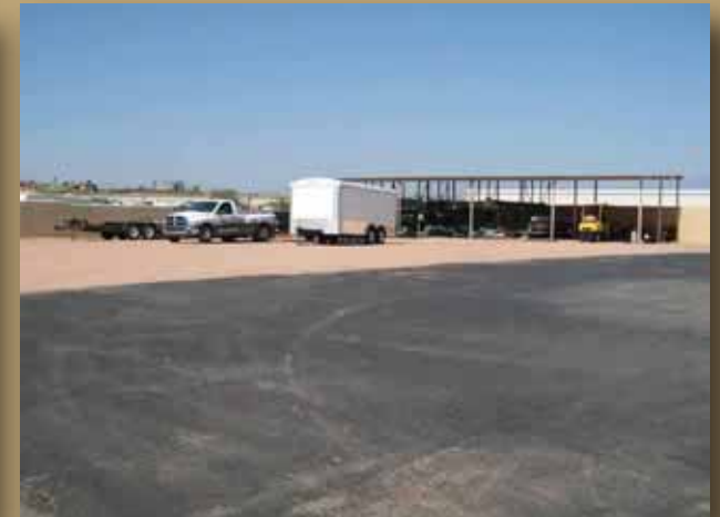
Private Fenced Yard with Carport
